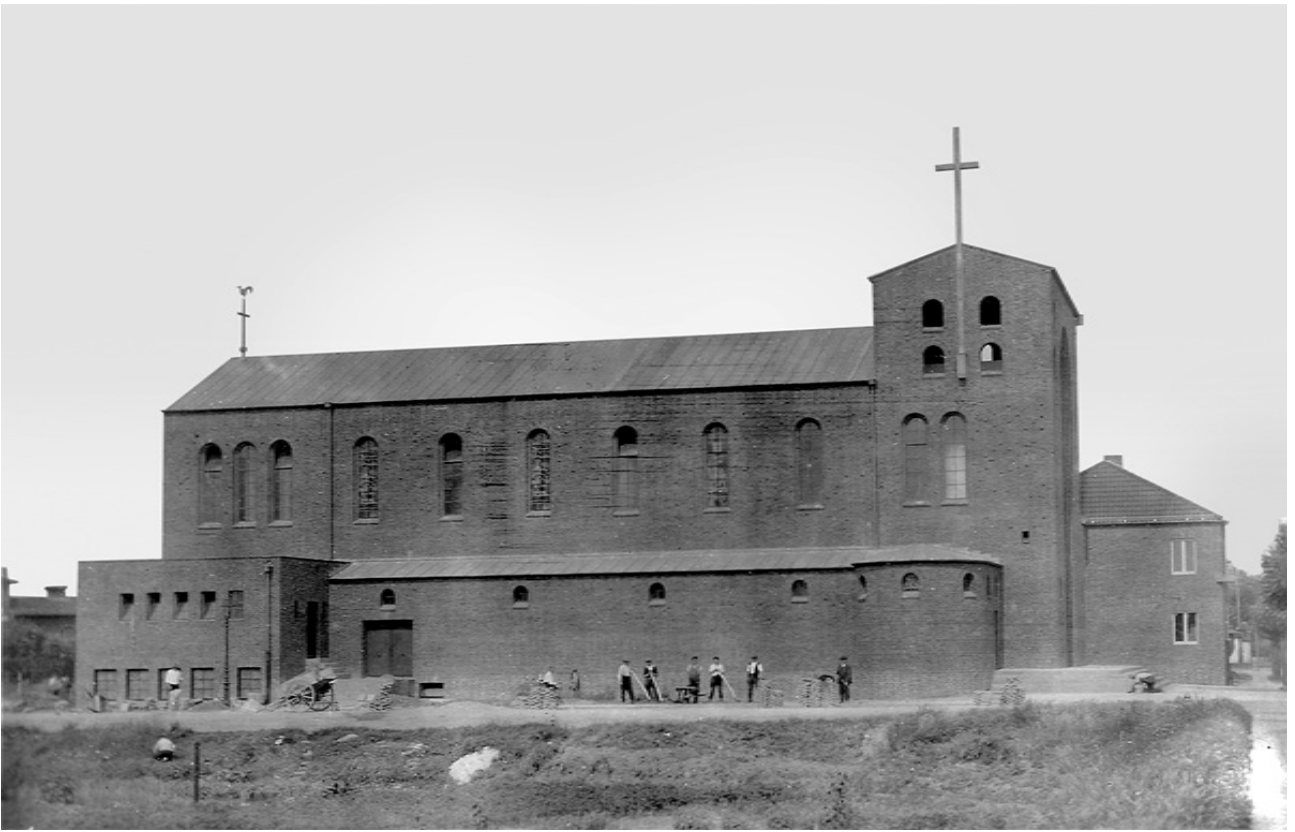
The new St. Barbara Church under construction, 1933
